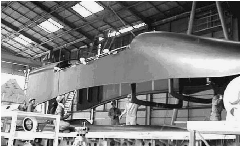
Figure 17. Coupling upper fuselage onto wing-body.
